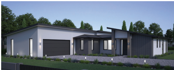
Style 2: Longrun mono roof with plaster, Linea and brick cladding
