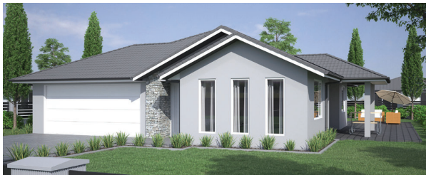
Style 2: Metal tile gable roof with plaster cladding
